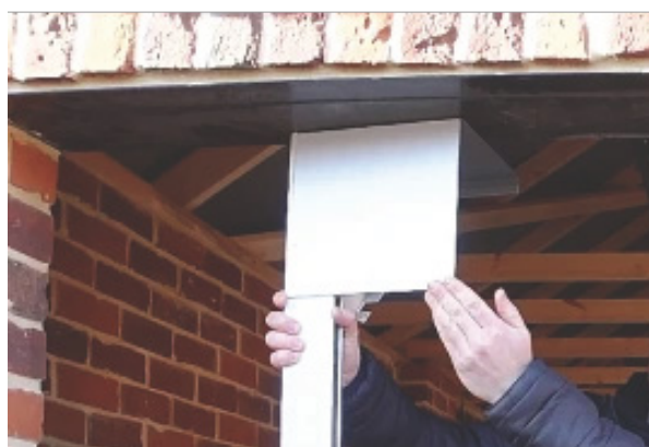
Top box beneath lintel
